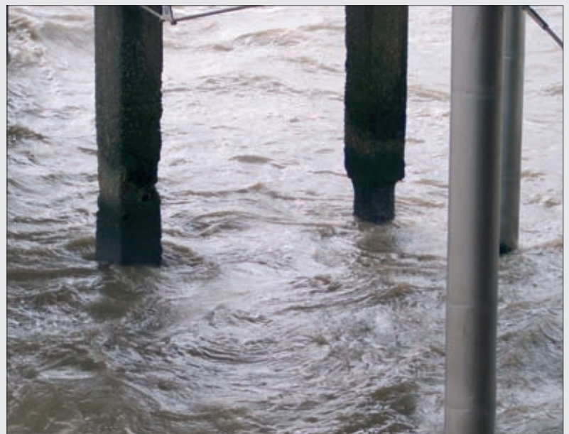
Heavily affected supports under the pier at Blankenberge (Belgium), a typical example of what happens if concrete is left unprotected.
