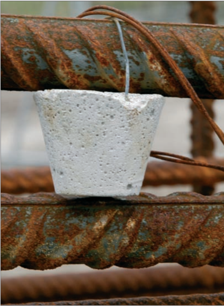
There is no need to derust reinforcing steel before the concrete is poured, since a very thin protective layer will eventually form that prevents the steel from corroding. Where things go wrong is when the protective layer breaks down.
