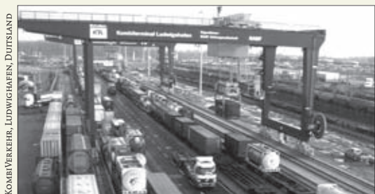
Road/rail terminal at Ludwigshafen, Germany. Existing road/rail terminals would offer the best candidates for the hub transfer technique, provided the cranes are supported by a local transport system. It may not even be necessary to use a robotic wheeled pallet system like the
