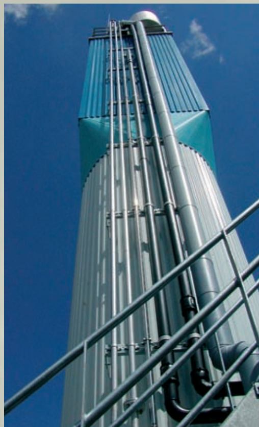
Rotterdam, Dokhaven. In the first industrial-scale Anammox reactor incorporating technology developed in Delft was started up. The installation removes a large proportion of the nitrogen from the waste water produced by the city of Rotterdam. The operational costs are only ten percent of what a conventional reactor would cost, and the Rotterdam process uses considerably less energy.
